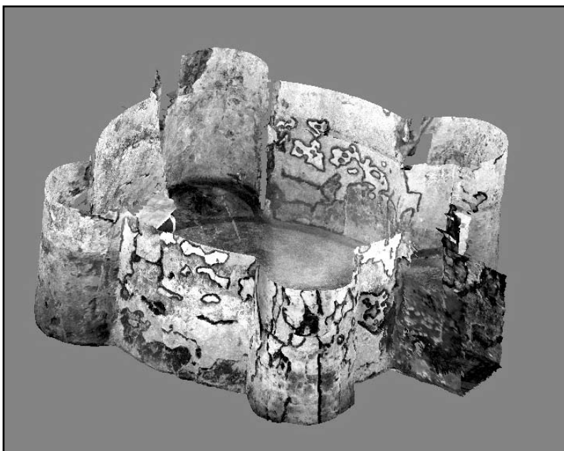
Cutaway view of 3D model of small room in the Suburban Baths by the ancient seashore of Herculaneum. The baths are where the first scanning efforts were concentrated because they’ve had to be closed to the public due to the deteriorating condition of the structure.
