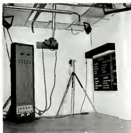
Fig. 1-4b: Fishing line-connected 3-D digitizing handle ("wand") resting on tripod (from [20])
