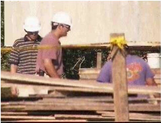
Construction Site Video
