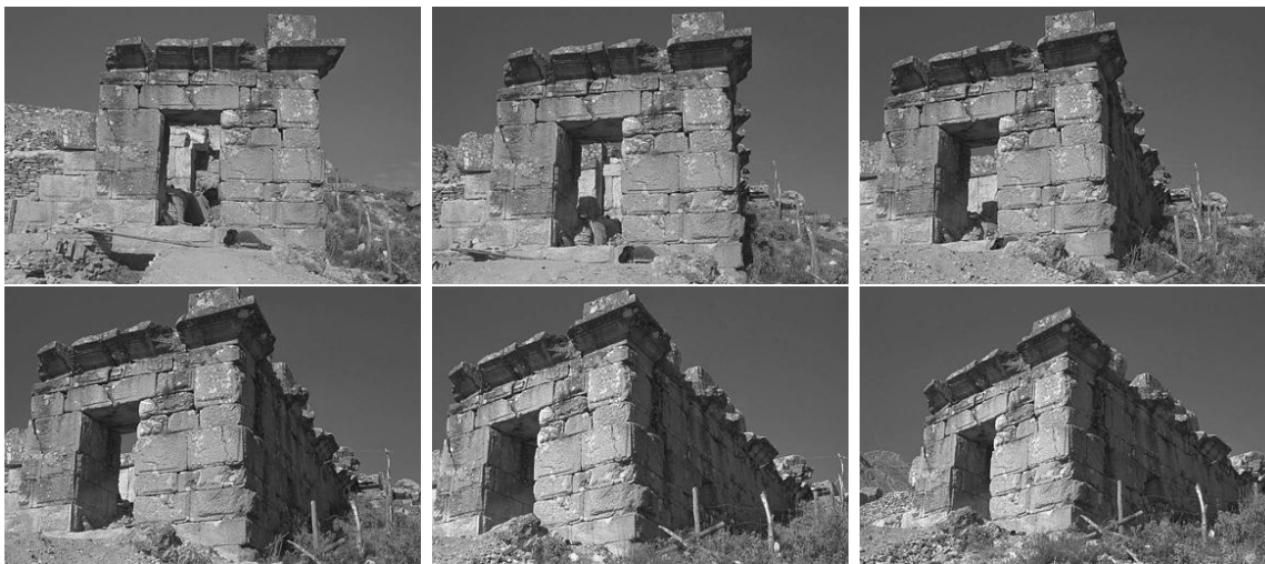
Figure 1: Image sequence which was used to build a 3D model of the corner of the Roman baths
