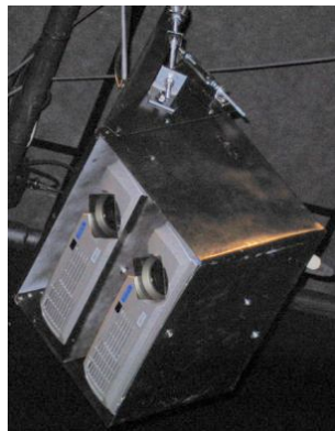
Figure 2: Projectors are mounted to the rack that is hanging from the ceiling.
